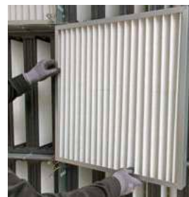
Easy replacement of pre- and main-filter
