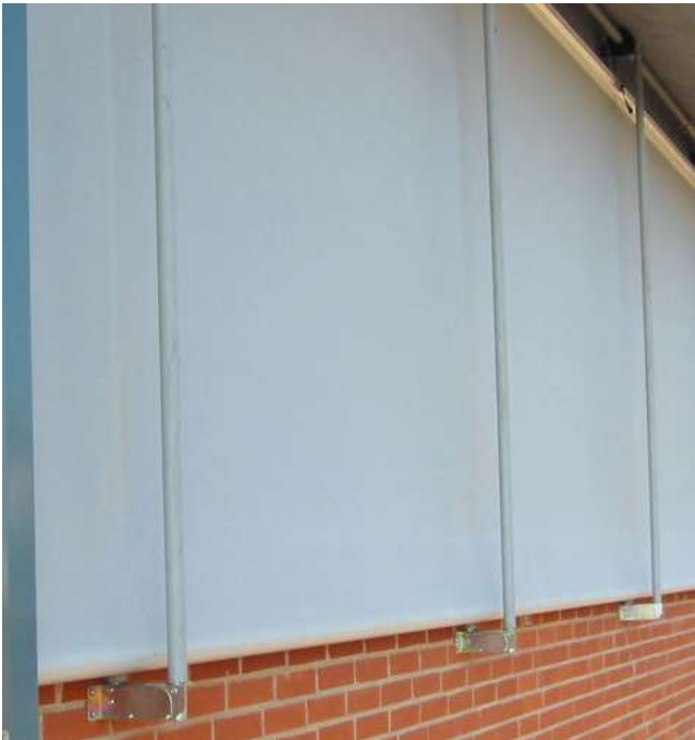
MSC wind protection pipes set
