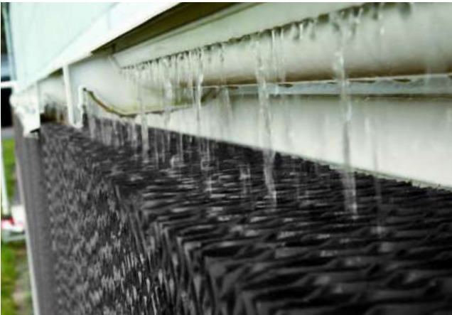
Water distribution in the Pad-frame system
